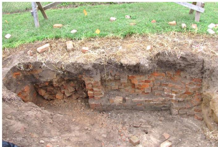
Part of the west foundation, collapsed fireplace base at left. Note under-fired salmon-colored bricks (interior of wall) and better-fired (darker) bricks.
