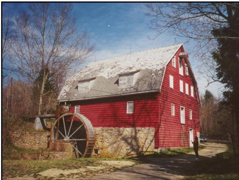
The mill is a four storey structure which has red siding today. There are two dormers on the side of the roof facing the river while the other side has three dormers. The millstones were on the second floor of the mill. The stones were driven by power from a twentyfoot diameter wooden overshot waterwheel. Today, the mill has a twentyfoot metal Fitz overshot waterwheel. All of the mill equipment has been removed. There is a metal pipe flume that directs the water to the wheel.
