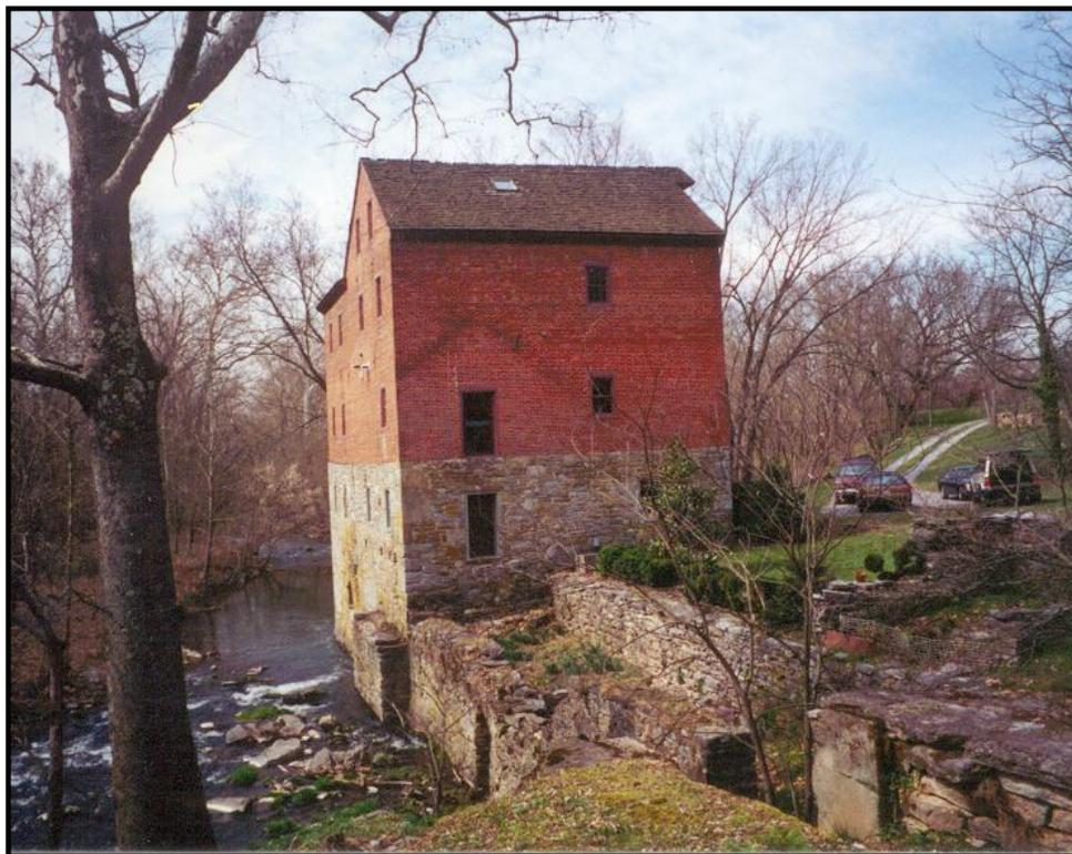
Aaron C. and Emory A. Pry were the owners of this mill in 1887. This was a four and a half storied brick mill that was built on a two storey stone foundation. The mill was set in a deep hollow on Upper Bridge Road. Also at this site was a cooper shop.
