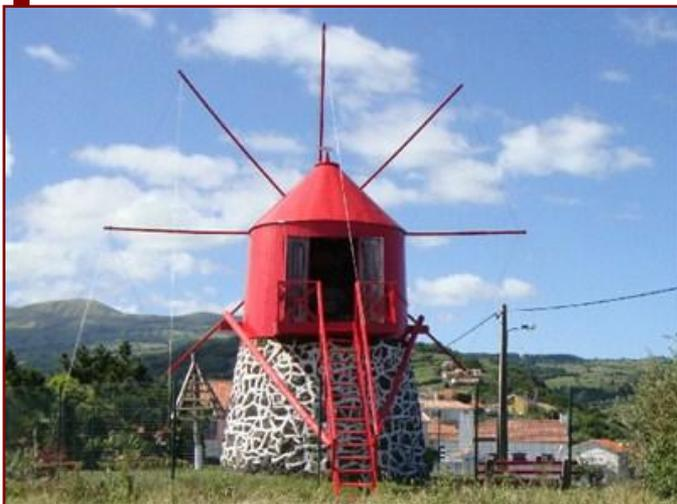
◀ On the islands of Faial and Pico, mills have a truncated cone-shaped stone base with a rotating wooden tower and central staircase that acts as a stabilizing “tail.” There is a central mast projecting outward to which 8 poles are wired so as to support triangular sails.
