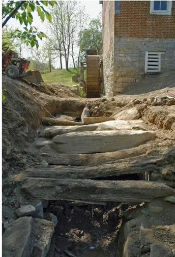
Later we had a surprise. Part of the bridge which supported the old gravel road which passes over the tail race, collapsed and allowed gravel and soil to fill the tail race. The nature of the bridge could not be seen until we excavated above it, and found large flat lime stones laid across the stone walls of the sides of the tail race.
