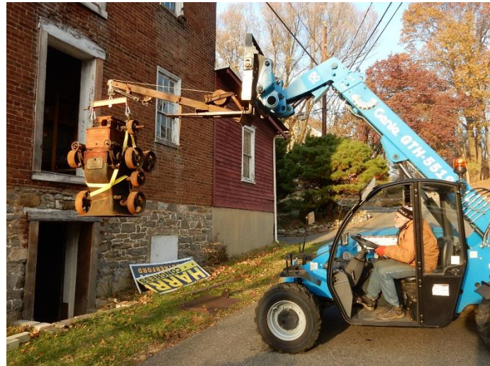
Photo 3: Reb Scavone's skill in handling the forklift and the fork-mounted crane that he designed were key to safely removing the roll stands from the second floor of Hawk Mill.
