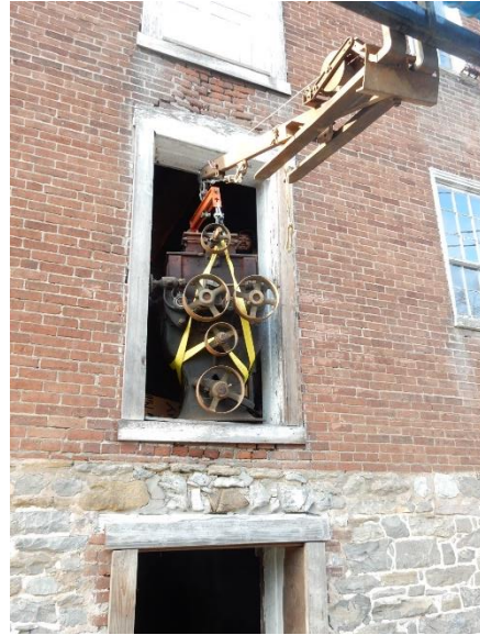
Photo 2: Both horizontally and vertically, the clearance was very tight.
