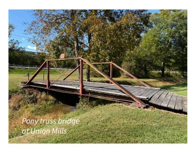
ed a few hundred yards from the original setting to its present site for use as a footbridge. According to historicbridges.org, it is an exceedingly rare example structure associated with famous civil engineer Wendel Bollman. Noted for its cast iron elements, the 3-panel, pin-connected, queen post bridge is called pony truss because the structure is not tall enough to have overhead cross-bracing, unlike a through truss bridge.
