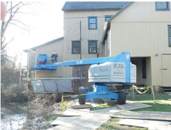
Figure 1 On the dam side of the mill, battens have been replaced where necessary, a door is being replaced, and painting is underway.
