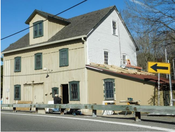
Figure 1 On the dam side of the mill, battens have been replaced where necessary, a door is being replaced, and painting is underway.
